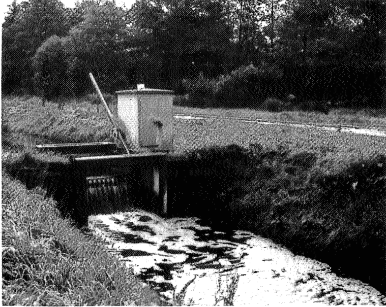
figure 6 Movable weir to maintain the water levels
